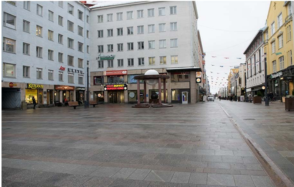
Figure 3. The heated pavement of the pedestrian street keeps the walking conditions similar all year round. The surface eases walkers and strollers to access the street in all weather conditions yet it is aesthetically poor (Oulu). (Source: Essi Oikarinen)
