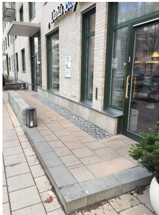
Figure 5. The standard requirement to create a level difference between the entrance level and the street level is an underlying factor, resulting in a special solution, separating people at the entrance. Still, there is a clear possibility to create an equal solution by bridging the level difference with a ramp inside the store.
