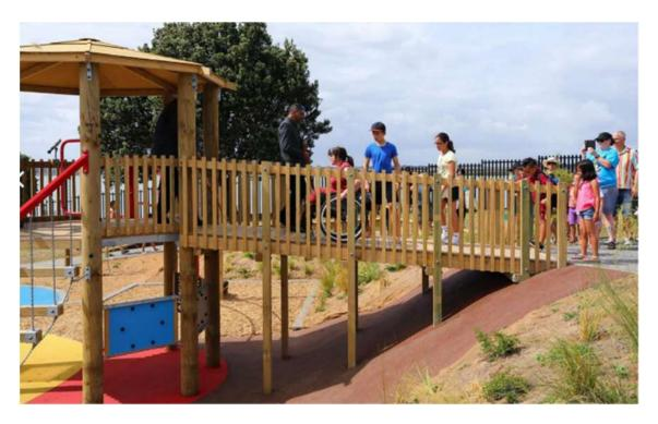
Figure 13. Gentle gradient ramp to the play tower.
