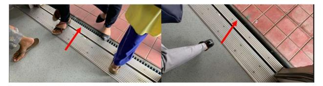
Figure 2. Different gap textures on Metro Line I. On the left, four people walk across the gap between the car and the station platform that has a small tooth-combed insert to bridge the gap. On the right, another station has a small gap (less than 5cm) between the car and the platform. Red arrows point to these features and illustrate the variable gap textures between cars and platforms at stations. Image Source: Sara Rotenberg.
