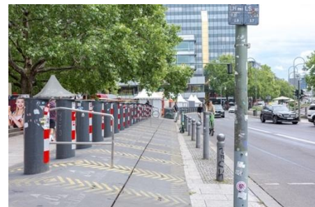
Figure 10. Hostile vehicle mitigation barriers
