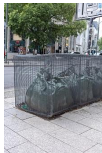
Figure 9. Sand bags as vehicle barriers
