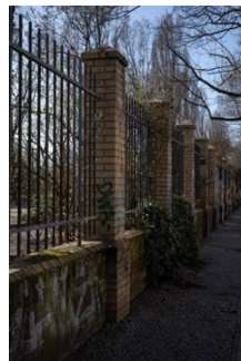
Figure 5. Perimeter wall on Görlitzer Str
