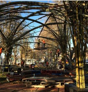
Figure 4: Roofing complete on central bay (left) and end bay (right). Images: Helen Norrie.
