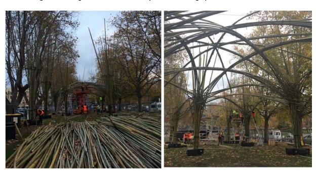
Figure 3: Central bay of canopy (left) and column and beam junction (right). Images: Helen Norrie.
