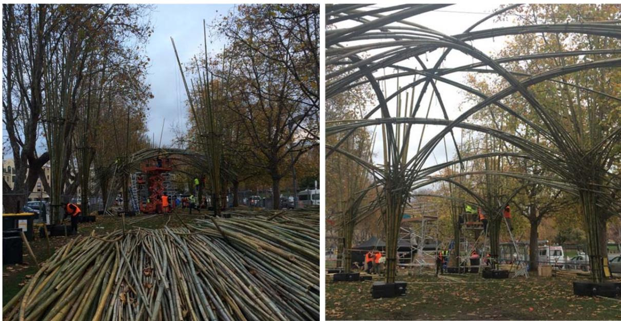
Figure 3: Central bay of canopy (left) and column and beam junction (right). Images: Helen Norrie.
