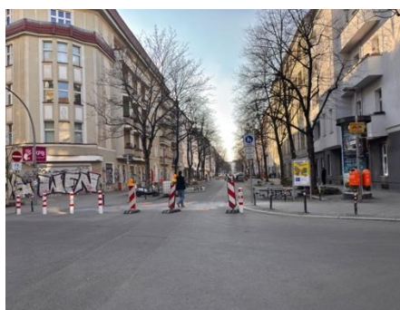
Figure 12. Access to Scharnweberstraße
